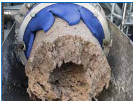
Paper mill - Pulp & paper (SEPCOM Industrial Horizontal)
